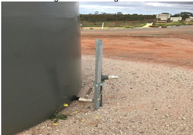
Photo showing Isolation valves on feeder main and filling pipe
