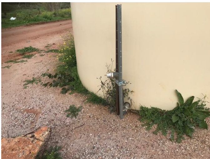
Photo showing Isolation valve on filling pipe
