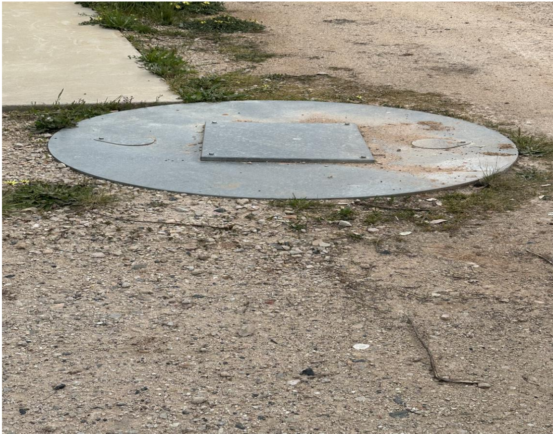
Underground septic tank
