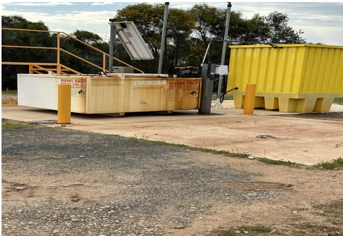
Self-bunded diesel tank
