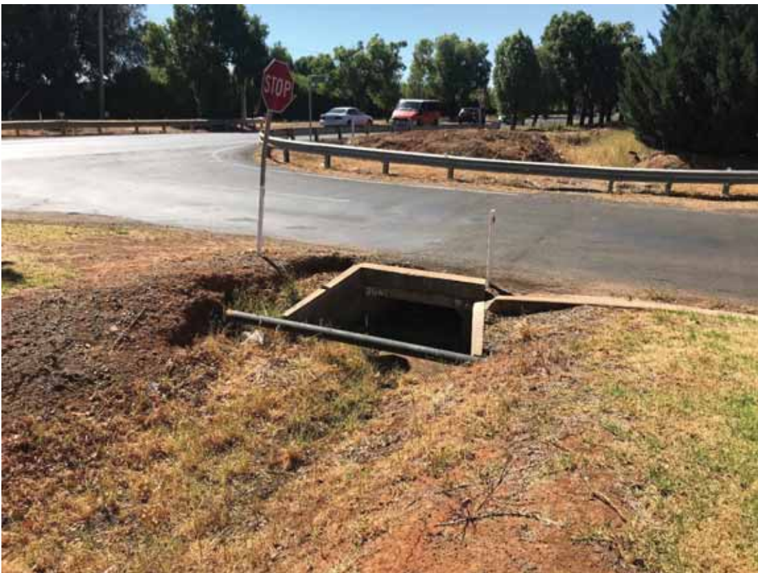
Figure 2-5 Box Culvert Under Leonard Road (Looking North)
