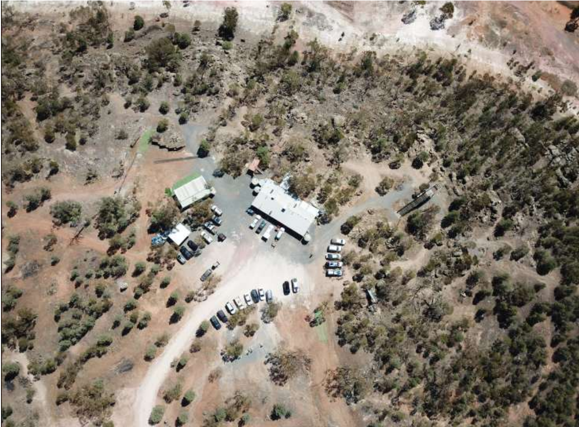
Figure 15: Aerial view of Clay Target Club
