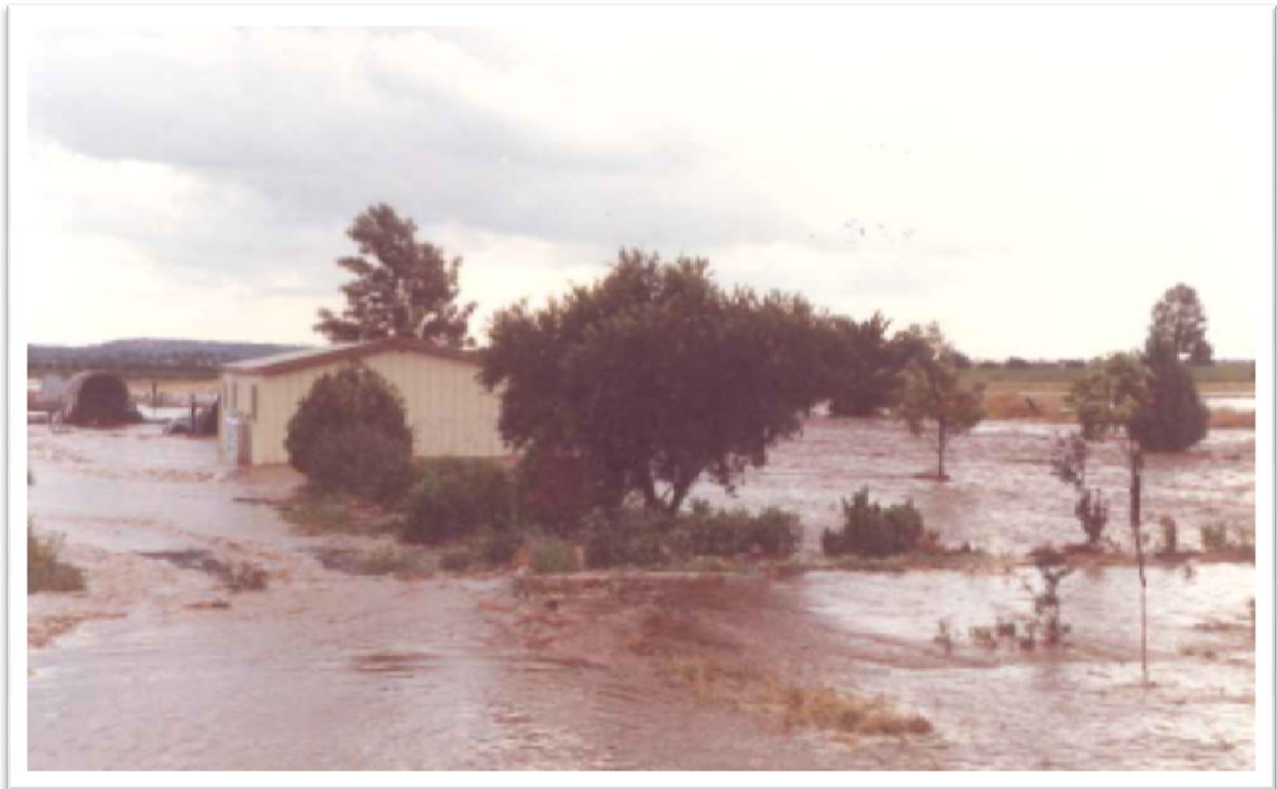
Figure 6-18 Flooding at Druit Road (March 1985)
