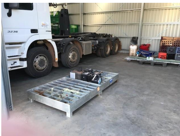
Figure 4.25: Bund for battery storage in the landfill workshop.
