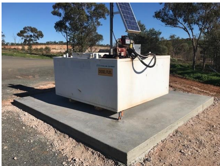
Figure 4.24: Concrete diesel fuel bund in an open area.
