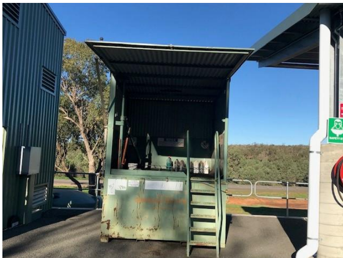
Figure 4.26: Bunded storage shed on site.
