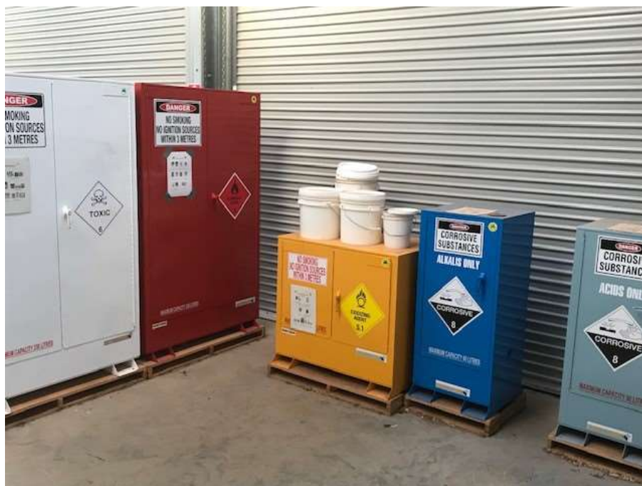
Figure 4.28: Chemical storage with signage within the landfill workshop.
