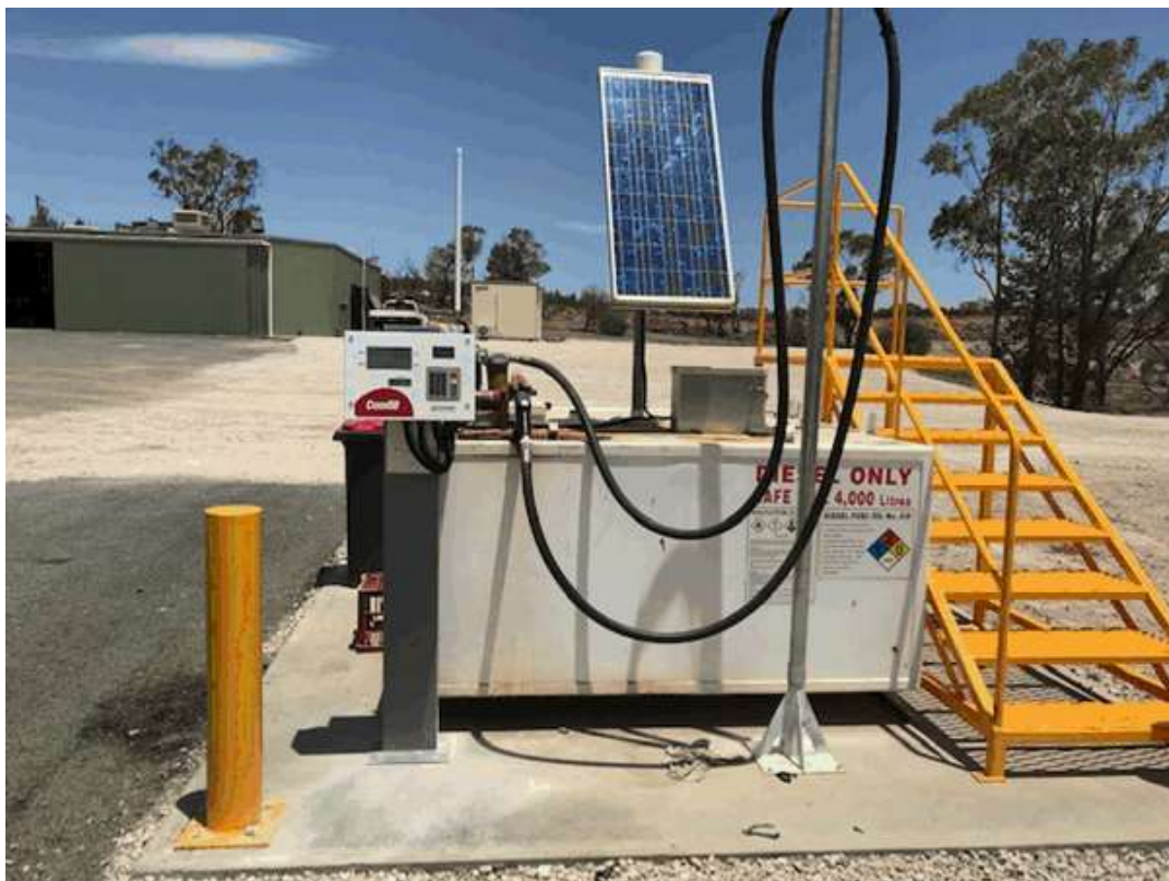
Figure 2.4: Newly installed diesel counter
