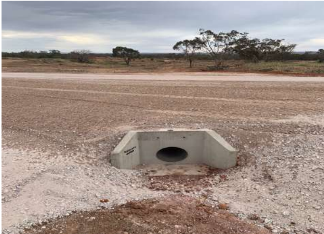
Figure 2.3: Stormwater pipes
