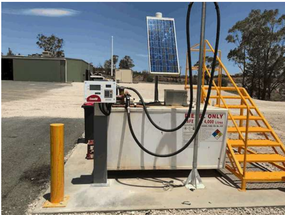
Figure 4.25: Concrete diesel fuel bund in an open area.
