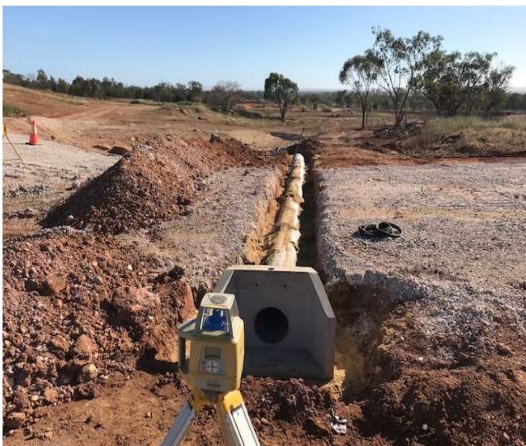
Figure 2.2: Construction of stormwater pipes
