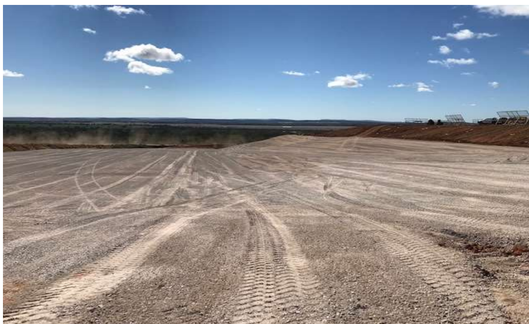
Figure 2.6: Completed landfill void cell floor
