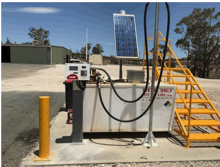
Figure 4.26: Concrete diesel fuel bund in an open area.
