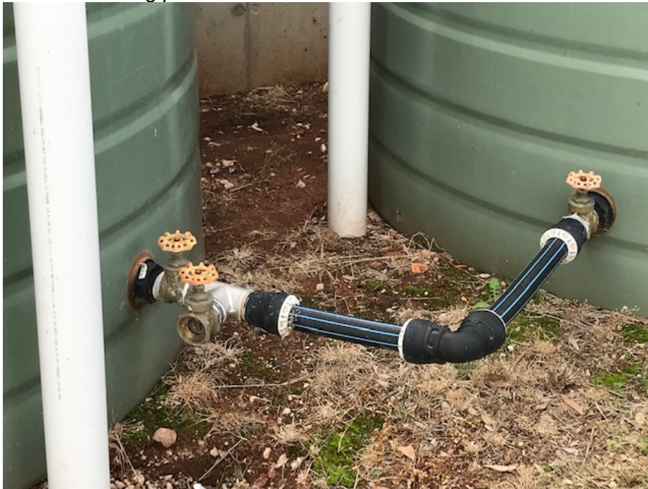
Photo of flushing point
