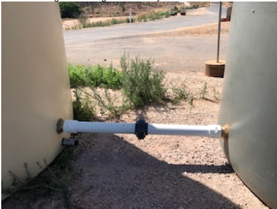
Photo showing tanks being connected by 100mm HD PVC.
