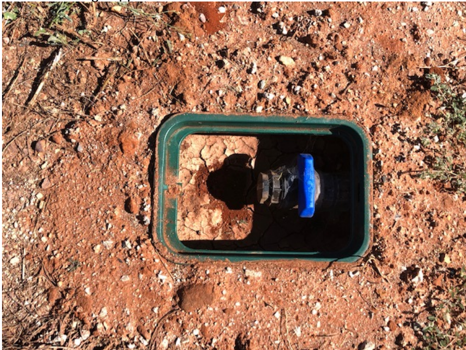
Photo showing capped water main
