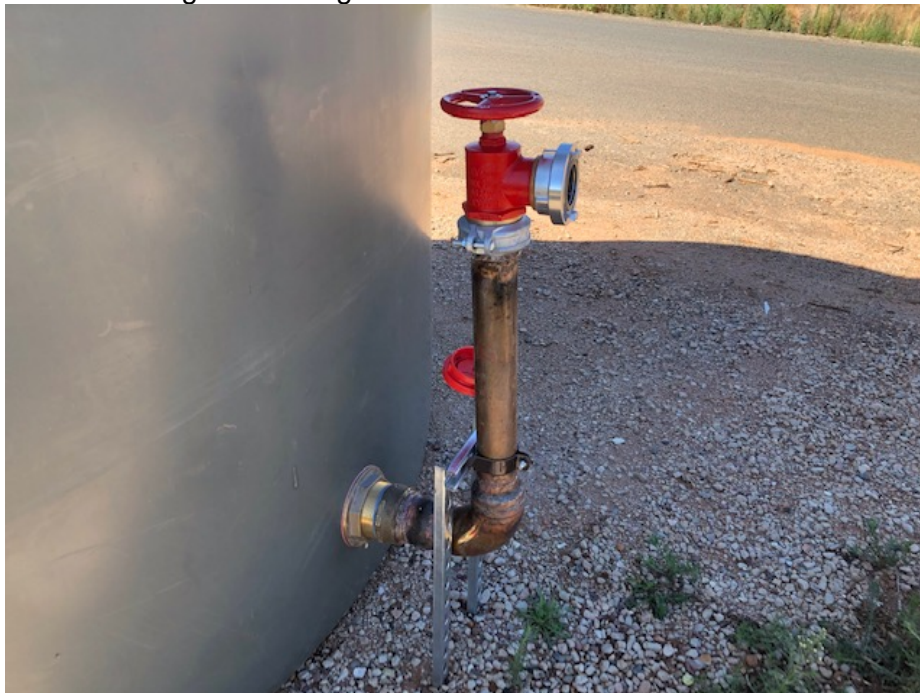
Photo showing Storz fitting
