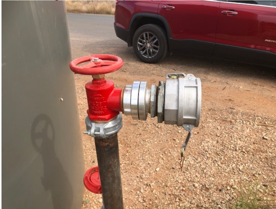
Photo showing Camlock fitting (female)
