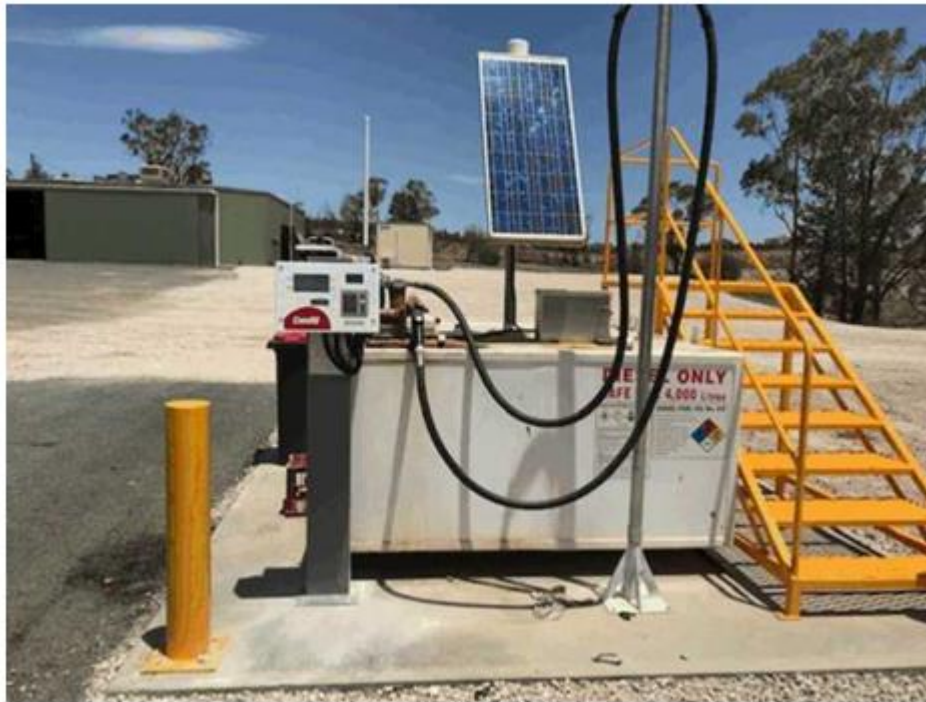
Figure 4-42: Concrete diesel fuel bund in an open area
