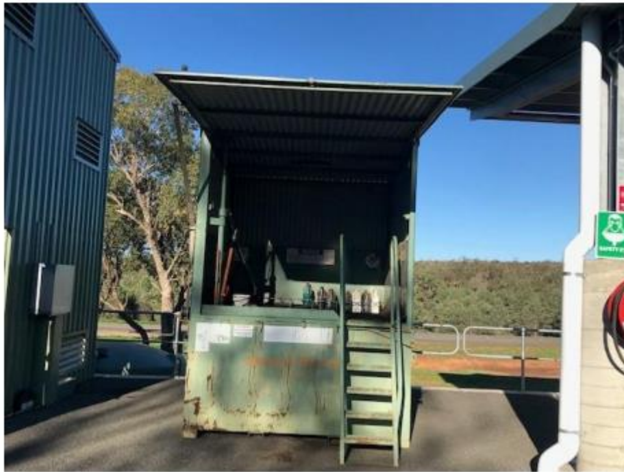
Figure 4-44: Bunded storage shed on site
